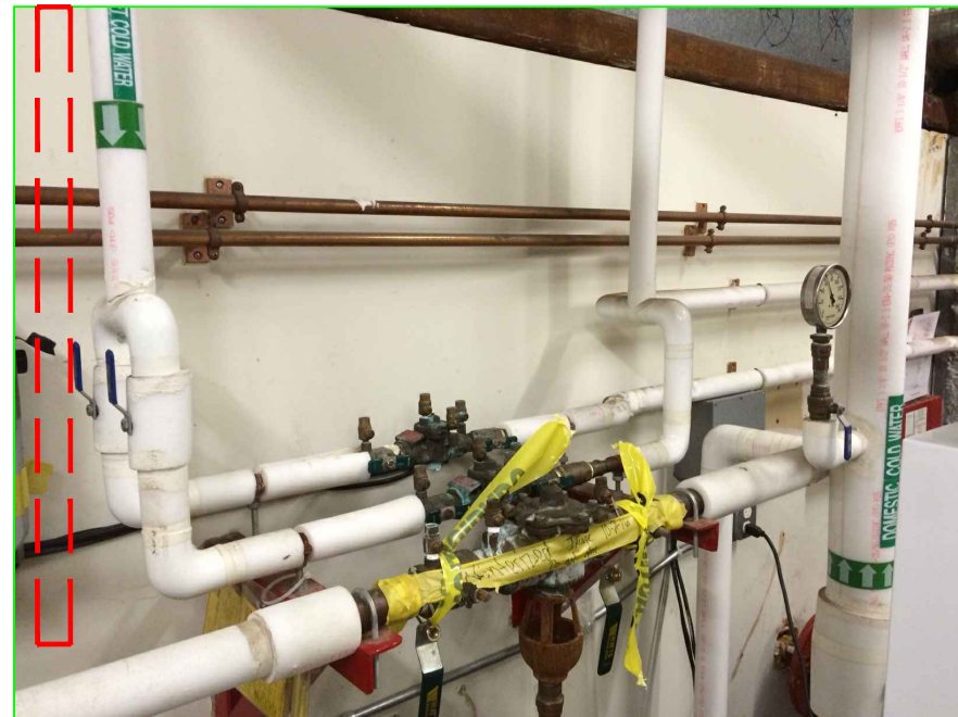
ROUTING UP FROM BUILDING ENTRY
