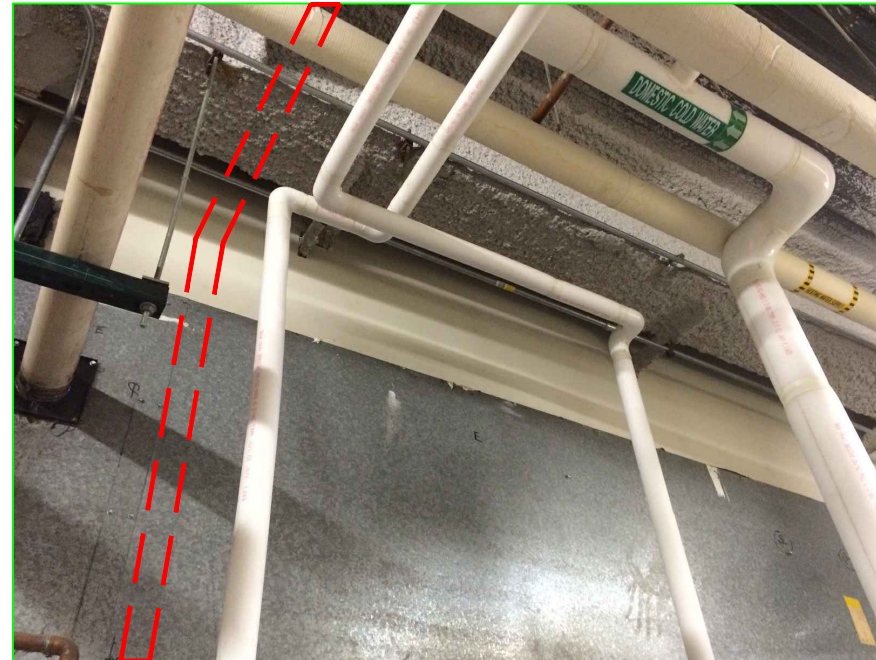
ROUTING UP FROM BUILDING ENTRY TO CEILING
