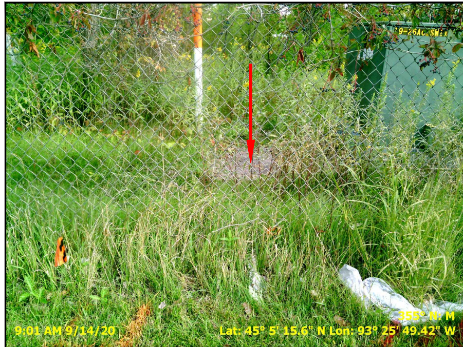
Existing Windstream HH
