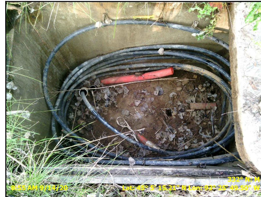
Existing Windstream HH
