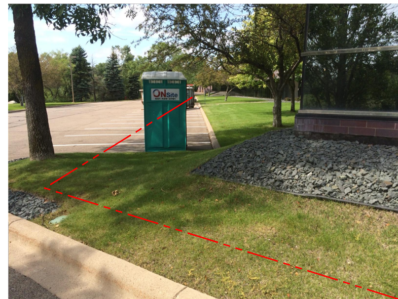
FROM HANDHOLE BORE UNDER PATHWAY, GRASSY AREA AND PARKING LOT, CONTINUE AROUND TO BACK OF BUILDING. 2 4
