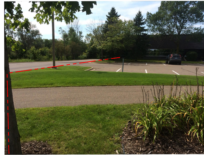
FROM HANDHOLE BORE UNDER PATHWAY, GRASSY AREA AND PARKING LOT, CONTINUE AROUND TO BACK OF BUILDING. 2 4
