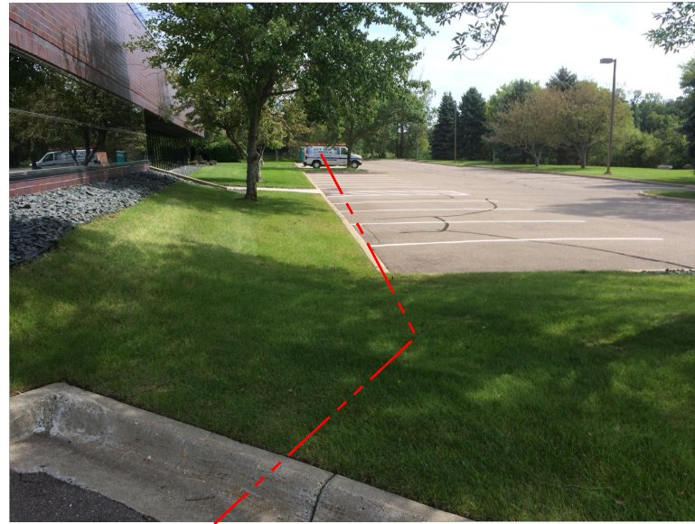
BORE BEHIND BUILDING. 5 4
