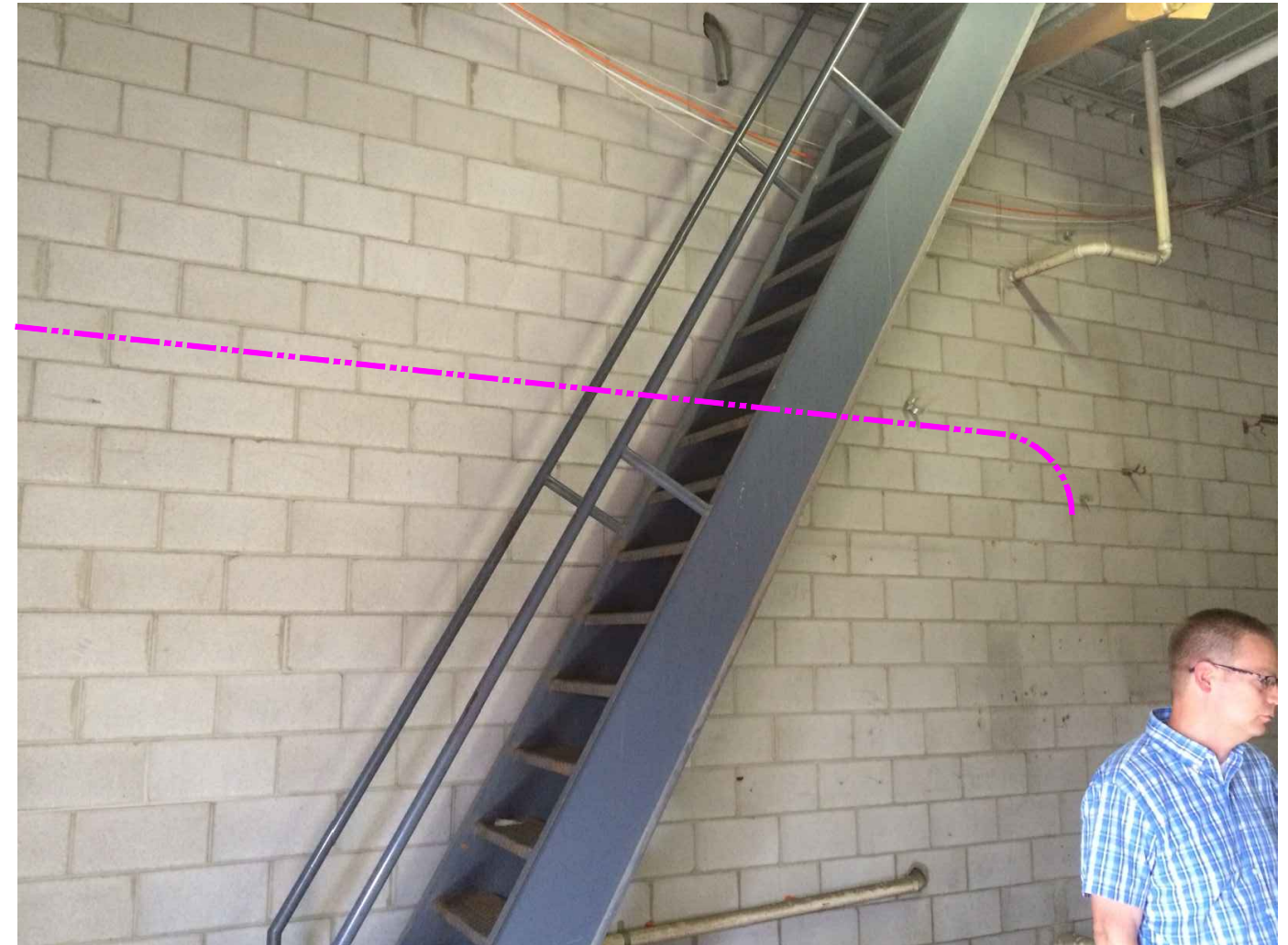
2" EMT ROUTE CONTINUING ALONG THE NORTH WALL PAST THE STAIR CASE TO THE BACKBOARD LOCATION.
