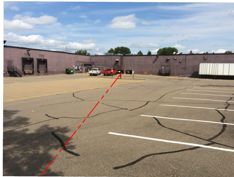
BORE UNDER PARKING LOT AT REAR OF BUILDING. 7 5
