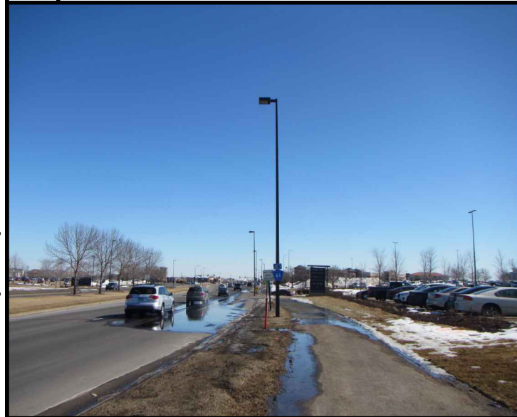
C OVERVIEW OF SITE
