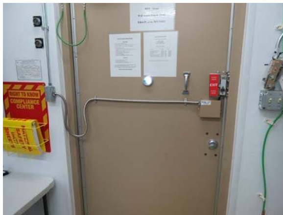
5 DOOR LOCK INSTALLATION PHOTOS SCALE: NONE
